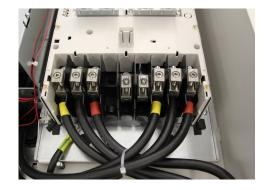
Connect the motor wires (from 1M contactor) to motor terminals of the drive.
