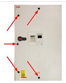
Rotate latches clockwise and open the enclosure door.
