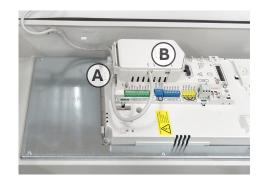
Using a PZ2 bit, loosen and remove wires from the input terminals of the drive.
