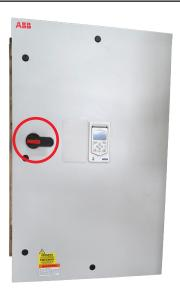
2 Rotate latches clockwise and open the enclosure door.
