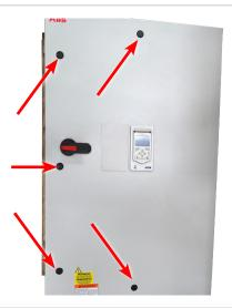
**3** Perform voltage check to confirm no voltage is present.
