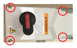
Remove covers and unclip the drive cover from the enclosure cover.
