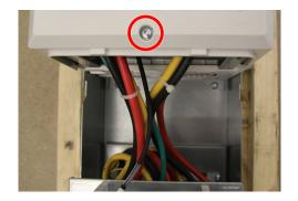
Using a T20 bit, loosen and remove one (1) M4x16 screws securing the inverter cover.
